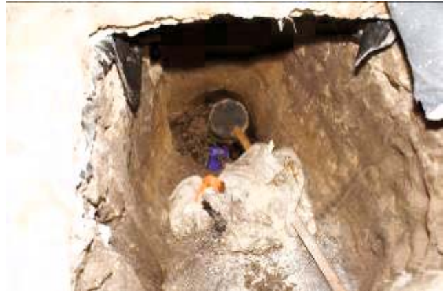
Waste dumped at the bottom of the hole and into the groundwater
