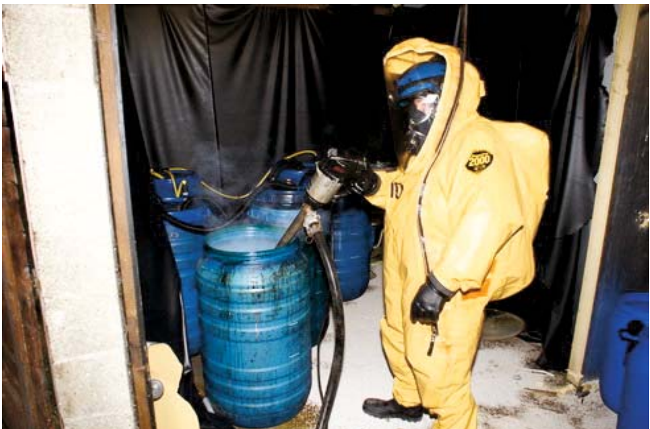
Dismantling in a Splash 2000 chemical suit
