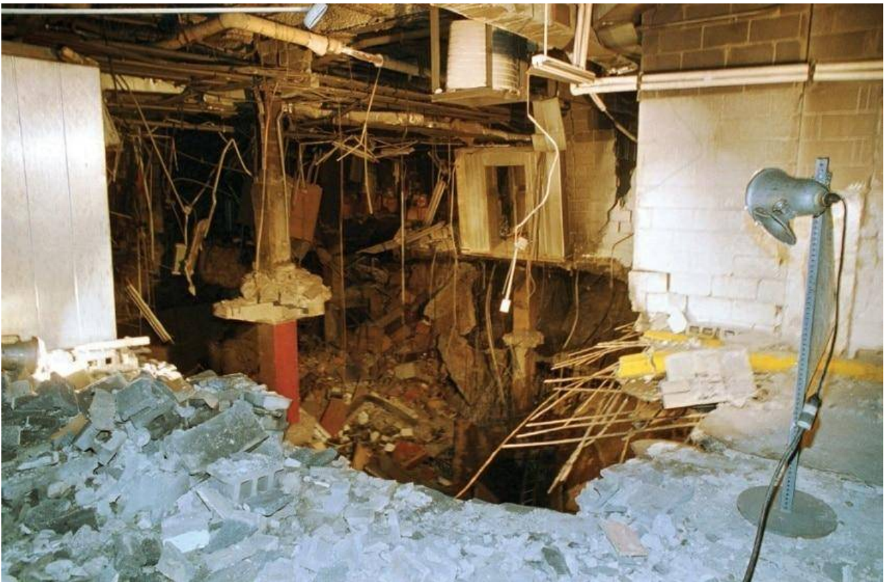
1993. New York City, New York. 6 killed, 1,042 injured. 606 kg urea nitrate. (Underground of WTC heavily damaged; building intact).
