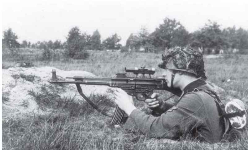
An MP 43/1 is tested at the Infanterie-Schule, Döberitz, in 1943. This weapon is fitted with a Zf 4 optical sight, although full-auto fire from the gun tended to knock the sight off zero. (BArch, Bild 146-1979-118-55, o. Ang.)
