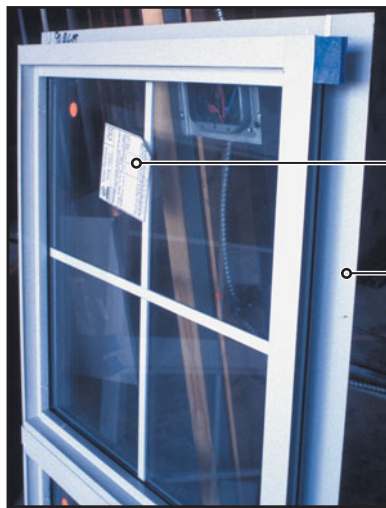
(a) A factory-glazed aluminum window with nailing flanges and simulated divided lites (muntins) within insulating glass unit
