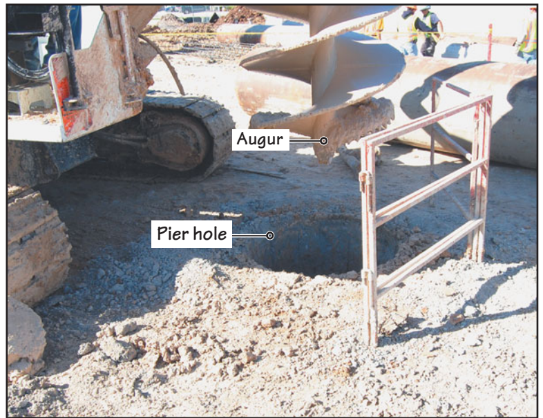
FIGURE 12.11 A typical auger for drilling a hole in soil.
