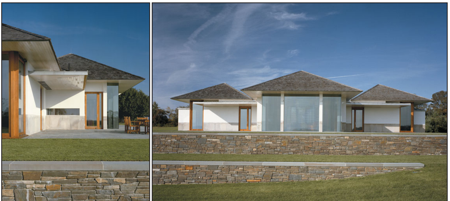
FIGURE 13.2 Millbrook Guest House in Millbrook, New York, by Meditch Murphey Architects—a wood light-frame house that takes advantage of natural ventilation, sunlight, and views. It is roofed with cedar shingles and clad with stucco and limestone base, with beech and teak used throughout the interior, courtesy of Meditech Murphey Architects. (Photographs © Maxwell Mackenzie)
