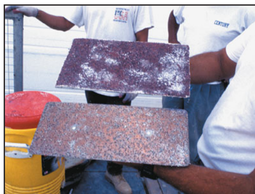
FIGURE 29.23 After the insulation has been adhered to the substrate, it is sanded smooth, a process called rasping . The right-hand lower photo shows two rasps with different roughness grades.
