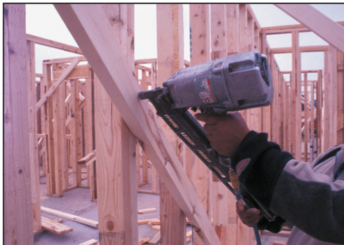
FIGURE 14.38 A typical nailing gun.
