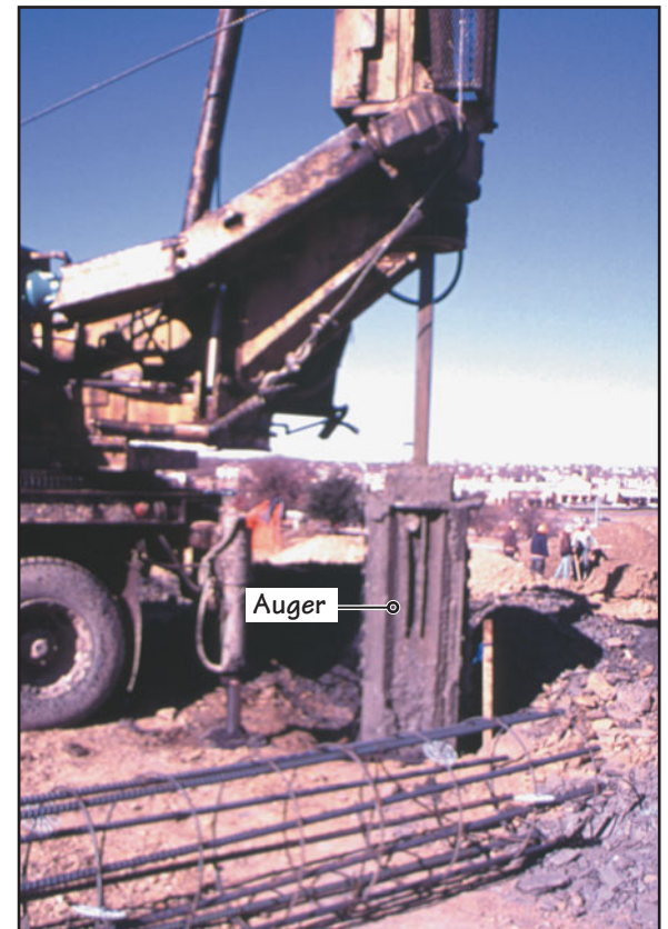
FIGURE 12.13 A typical bucket-type auger for drilling in soil.
