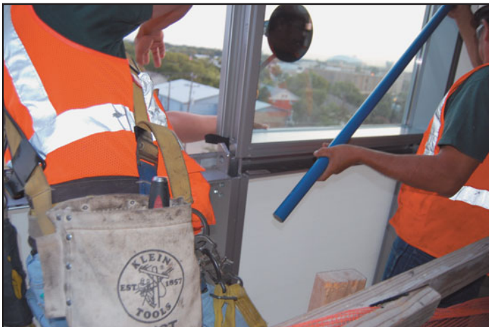
(c) The new unit being forced over the (projecting) splice
