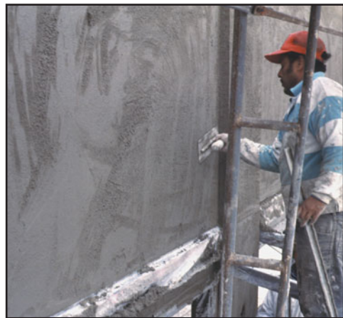
(b) Troweling the brown coat
