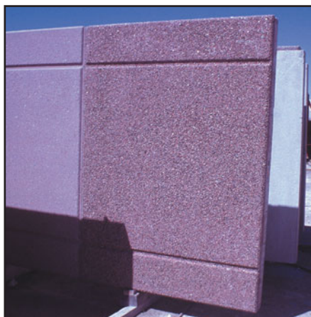
FIGURE 28.39 (b) The part of this panel on the left side of the reveal is lightly abrasive-blasted, and the right side part is medium abrasive-blasted.
