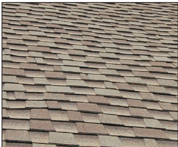
FIGURE 34.4 Asphalt shingles with color variations in their granule surface that give shadow lines to mimic wood or slate roofing.
