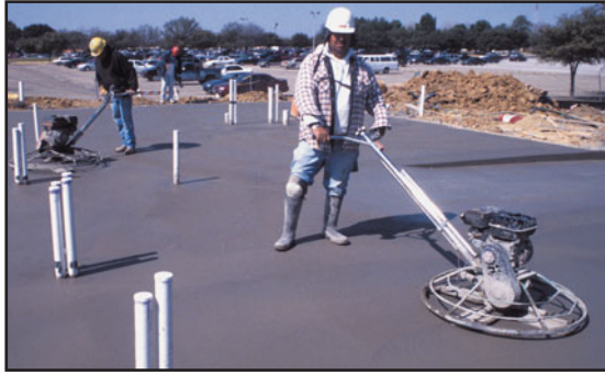
FIGURE 21.31 Troweling of concrete with a power-driven troweling machine, which is available in two different types, as shown. Each machine has metal blades that rotate over the concrete surface.
