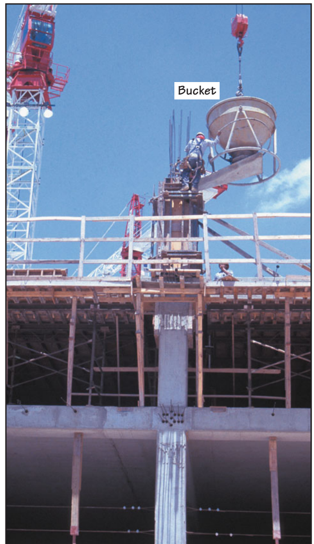
FIGURE 21.25 Concrete being filled in the bucket, which is hoisted into position using a crane. The bucket method of transporting concrete is generally used for small quantities of concrete, where pumping of concrete is uneconomical. Note that a large quantity of concrete is required to fill a pump line, which is wasteful if the quantity of concrete to be placed is small.
