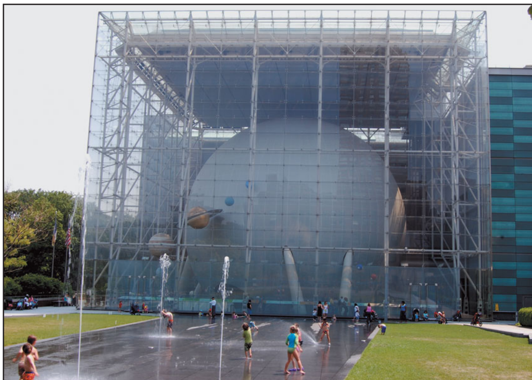
FIGURE 30.4 A transparent cube of glass, supported by a light steel structural backup, encloses the Rose Center for Earth and Space, New York City (see also Chapter 32, Figure 32.17). Architects: Polshek Partnership.
