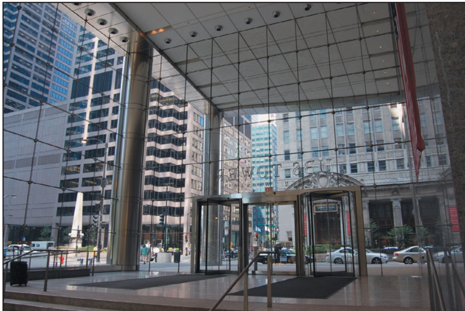
(a) Cable-net glass wall in the entrance lobby of the One North Wacker Building, Chicago, Architects: Goettsch Partners.
