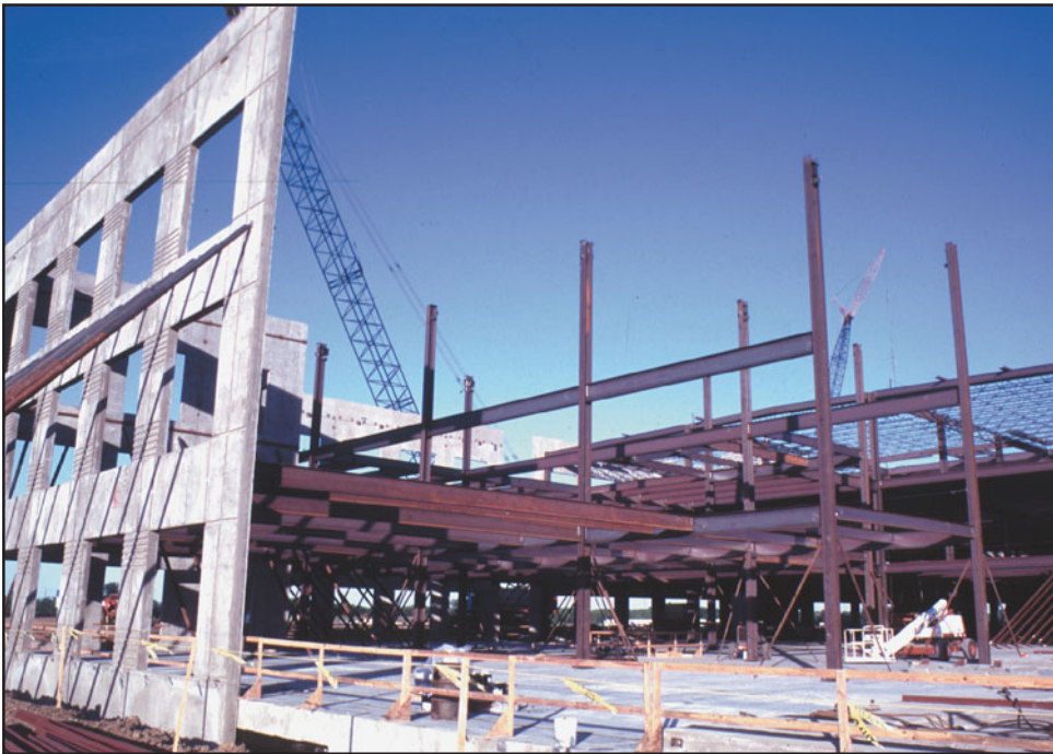
FIGURE 26.31 Most tilt-up buildings use tilt-up exterior bearing walls with an interior steel-frame structure.
