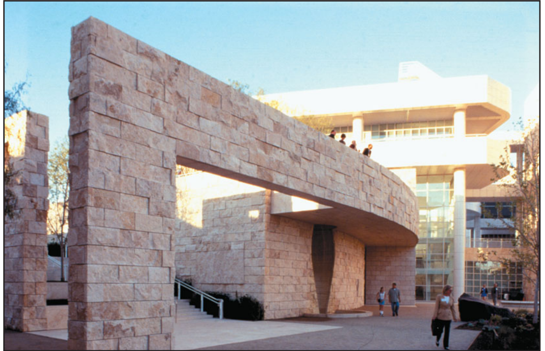
FIGURE 24.1 (a) Split-face (cleft) Italian travertine used as cladding material in the J. Paul Getty Center, Los Angeles, California (a complex of several buildings). The building in the background is clad with metal panels. Architect: Richard Meyer. (Photo courtesy of Dr. Jay Henry)
