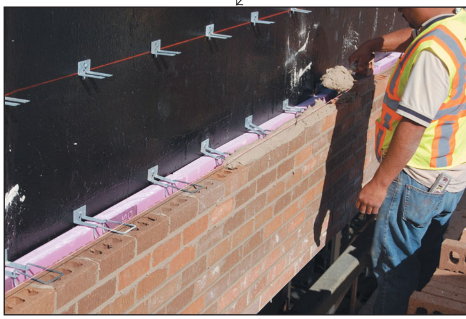
(c) A typical two-piece anchor consisting of a: (i) sheet metal anchor and (ii) wire anchor for reinforced-concrete backup members (walls, beams, and columns)
