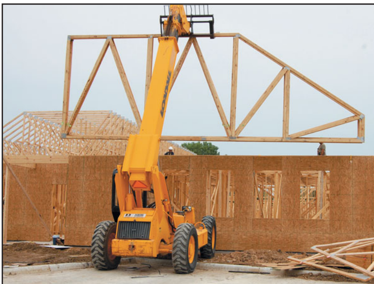
FIGURE 14.23 Because wood trusses are made from thin (2-by) members and connected together with (sheet steel) nail plates, they must be handled carefully during hoisting or placing in position so that the nail-plate connected joints do not open up. That is why, as shown in this figure, a roof truss is being carried in vertical alignment by a fork lift.
