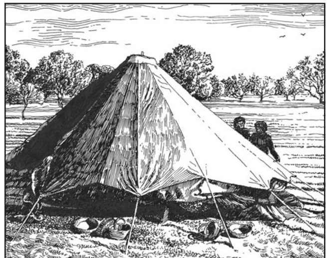
FIGURE 3.22 A tent resists earthquake forces admirably due to its light weight and its ability to absorb deformations.
