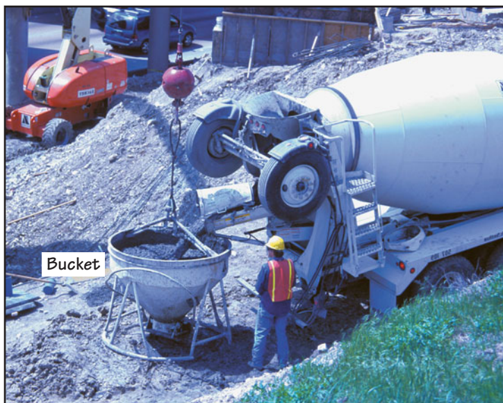
FIGURE 21.25 Concrete being filled in the bucket, which is hoisted into position using a crane. The bucket method of transporting concrete is generally used for small quantities of concrete, where pumping of concrete is uneconomical. Note that a large quantity of concrete is required to fill a pump line, which is wasteful if the quantity of concrete to be placed is small.
