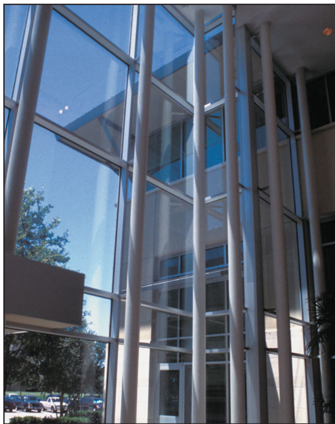
FIGURE 32.16 A tall glass wall with standard curtain wall sections anchored to an interior structural steel vertical member to provide lateral-load support to aluminum mullions. In this building, a steel pipe support is used. In taller walls, vertical steel trusses are common.
