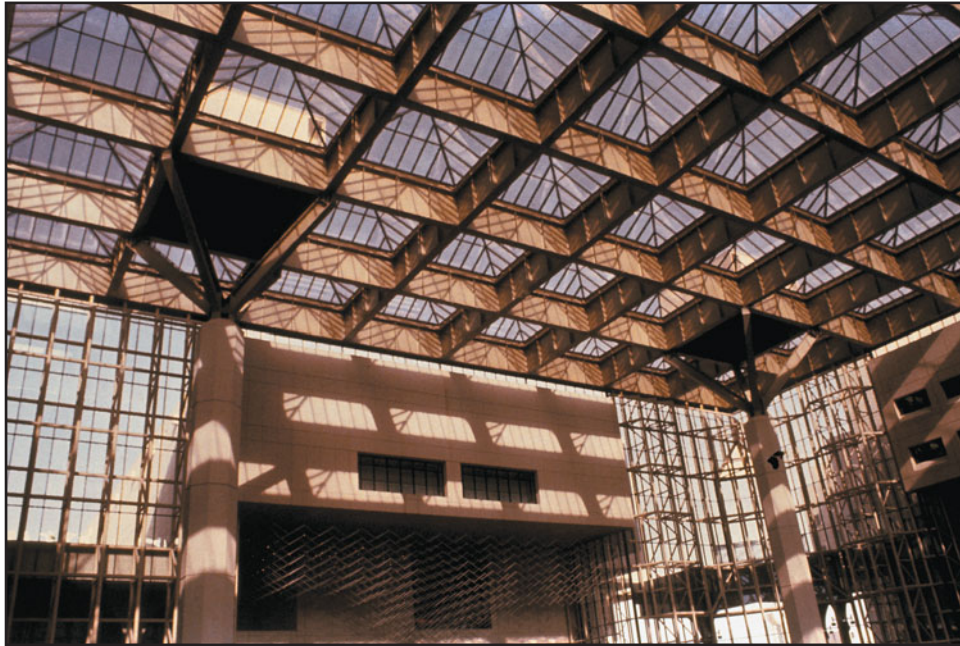
FIGURE 29 The roof of a large atrium space consisting of a two-way grid of W-shape beams, King Saud University, Riyadh, Saudi Arabia.
