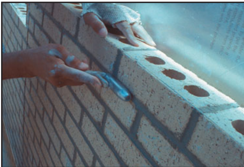
FIGURE 24.28 Steps involved in constructing a single-wythe brick wall.
