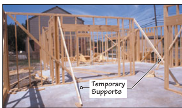
FIGURE 5 Wall assembly under construction.
