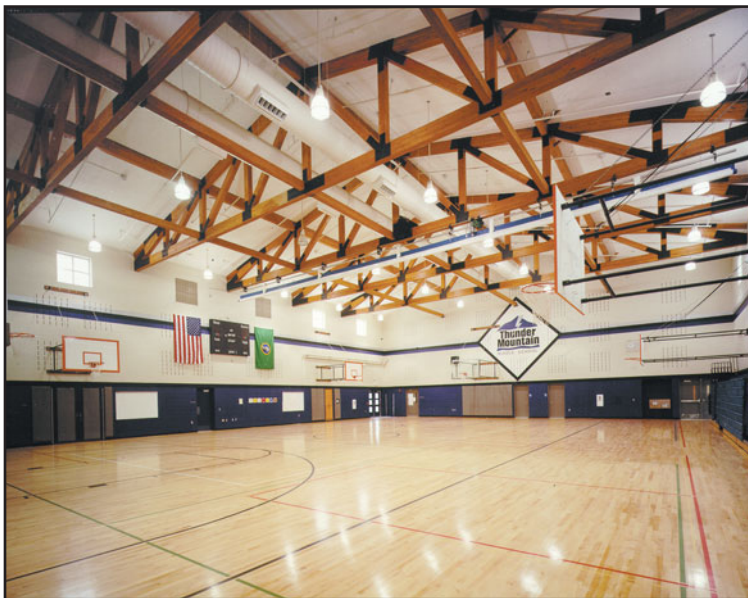
FIGURE 14.4 Glulam trusses used in the gymnasium of Thunder Mountain Middle School, Enumclaw, Washington. Architect: BLRB Architects, Tacoma, Washington. (Photo courtesy of APA—The Engineered Wood Association)
