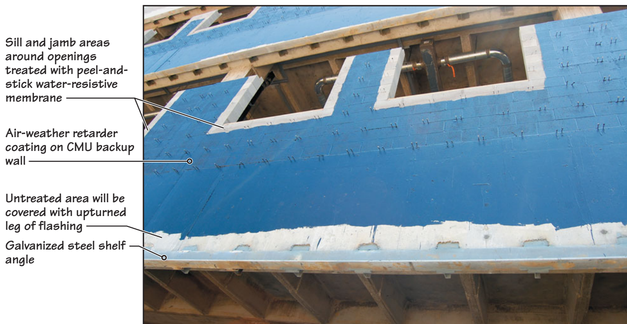
FIGURE 28.25 The exterior surface of a CMU backup wall (and the underlying spandrel beam) has been treated with a liquid air-weather retarder (blue color) before the brick veneer is constructed.
