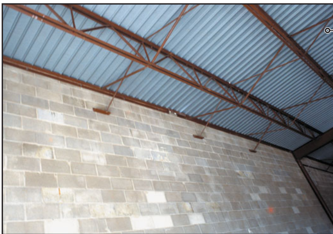
FIGURE 18.23 Diagonal bridging of steel joists is an alternative to horizontal bridging. Regardless of the bridging system used, the bridging members in the end spans must be securely connected to the exterior wall (as shown here) or the spandrel beam.
