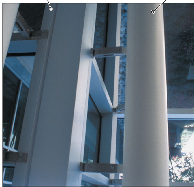
FIGURE 32.16 A tall glass wall with standard curtain wall sections anchored to an interior structural steel vertical member to provide lateral-load support to aluminum mullions. In this building, a steel pipe support is used. In taller walls, vertical steel trusses are common.
