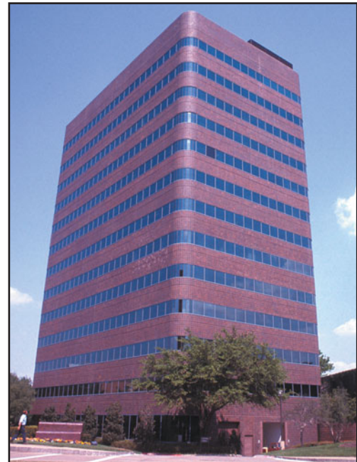
FIGURE 28.24 A building with brick veneer spandrels and ribbon windows.
