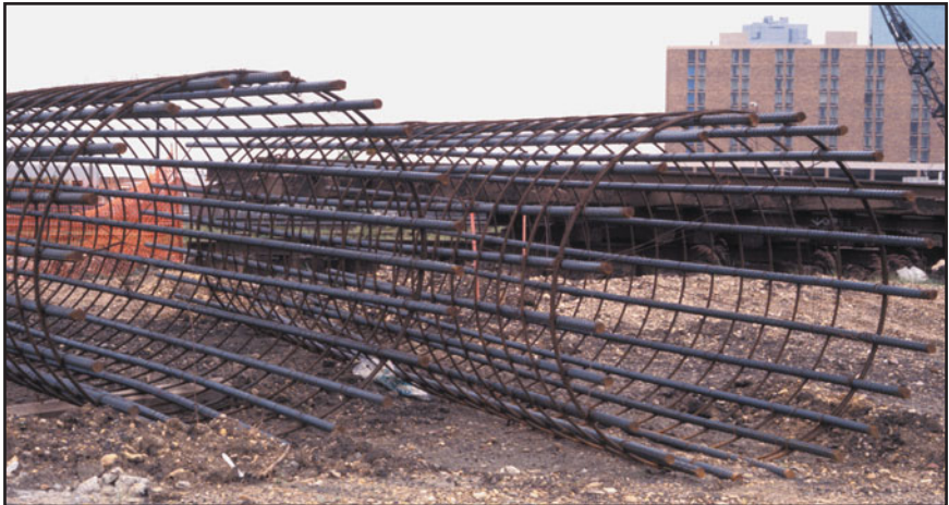
FIGURE 22.28 Reinforcement cage for a round column with circular ties.
