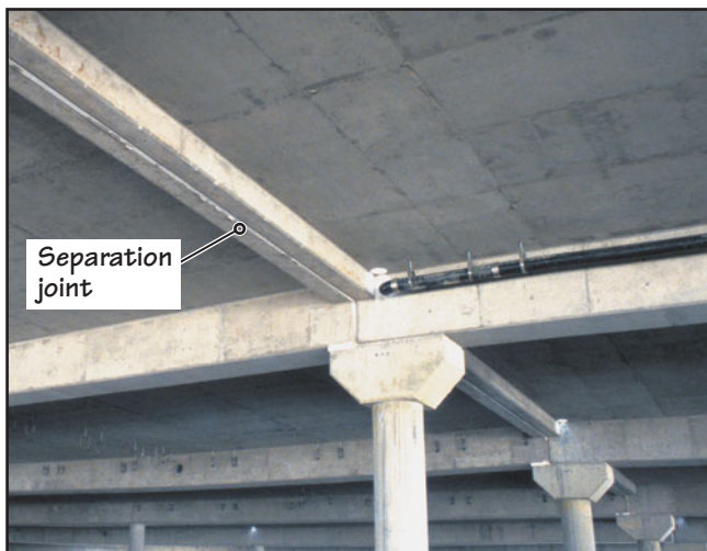
FIGURE 9.7 Building separation joint using a single column in a reinforced concrete building (see Expand Your Knowledge in Chapter 23 for details). Observe the provision of a beam on each side of the separation joint.
