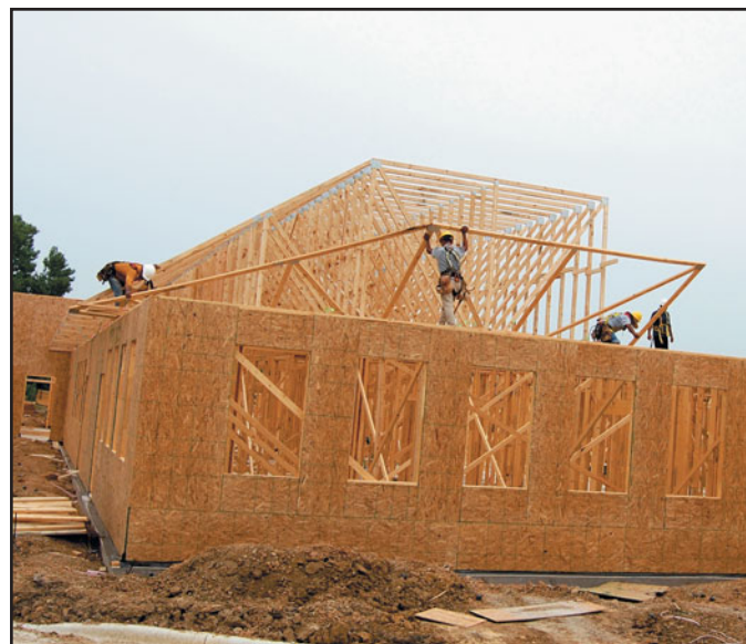
FIGURE 14.23 Because wood trusses are made from thin (2-by) members and connected together with (sheet steel) nail plates, they must be handled carefully during hoisting or placing in position so that the nail-plate connected joints do not open up. That is why, as shown in this figure, a roof truss is being carried in vertical alignment by a fork lift.
