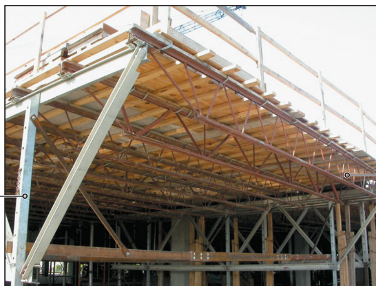
FIGURE 22.11 Details of the panelized flying form in Figure 22.10. The panel consists of steel joists that are supported on two aluminum trusses, one at each end. The vertical members of trusses extend down to form shores, which are provided with adjustable jacks. The steel joists support lumber planks, which in turn support plywood sheathing.
