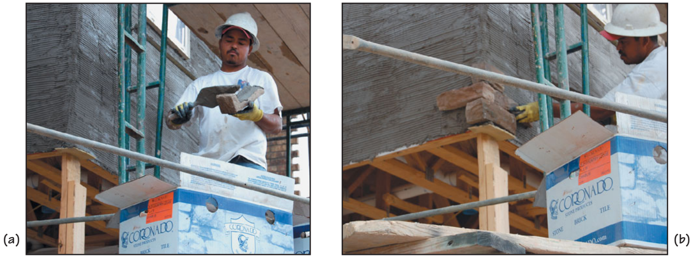
FIGURE 29.16 (a) A mason applying mortar to the back of a manufactured stone (corner) unit. (b) Masonry unit being adhered to a scratch-coated wall surface.
