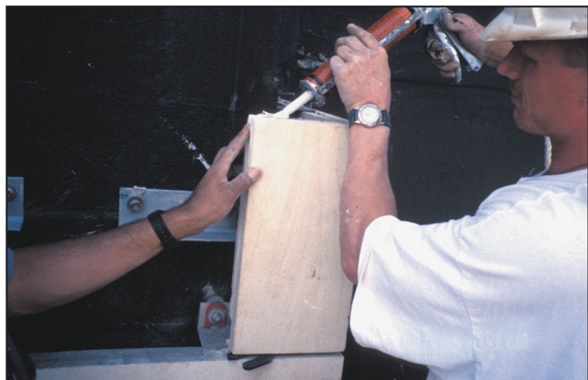
FIGURE 29.37 Applying sealant in kerfs of a stone slab before inserting tiebacks.
