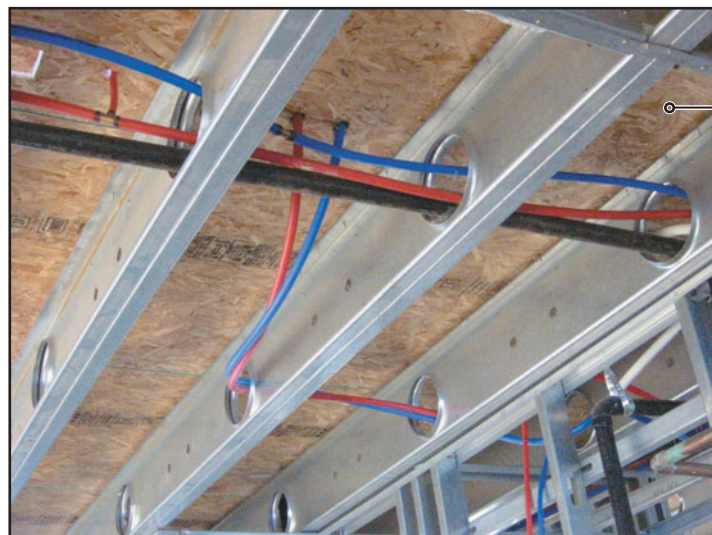
FIGURE 20.24 CFS floor joists with extruded holes allow utility lines to pass through. (Photo courtesy of Dietrich Metal Framing)
