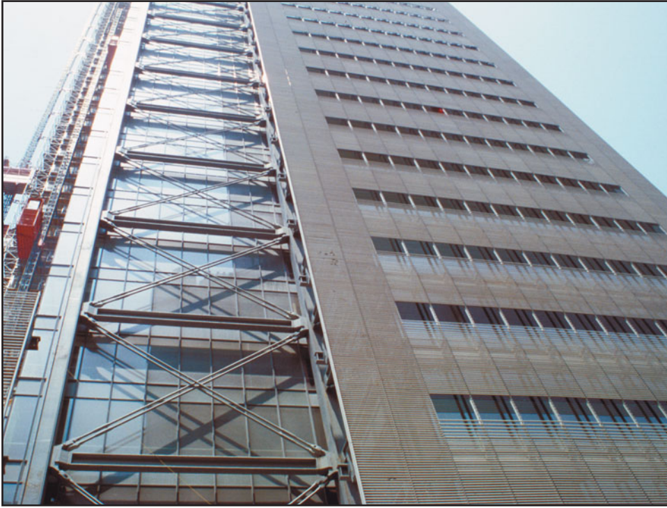
FIGURE 3.8 Diagonal braces used on the exterior facade of the 52-story New York Times Building, New York City, provide lateral load resistance. The building was designed by Renzo Piano Building Workshop in collaboration with Fox and Fowle Architects and was completed in 2007.
