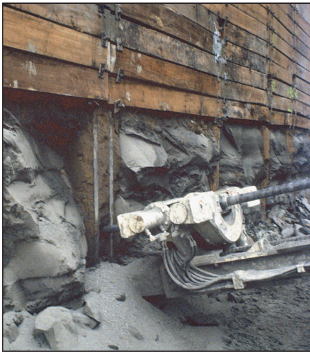
FIGURE 11.18 (a) The hole for a tieback is drilled through the space between the twin steel channels comprising the pile. (b) A high-strength steel tendon is now placed into the hole, and the hole is filled with portland cement-based grout. After the grout has gained sufficient strength, the tendon is stressed to the required tension and anchored to the pile as shown.
