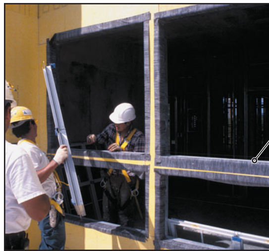
(b) Window being brought into the opening. Observe the self-adhering waterproof tape around the rough opening.
