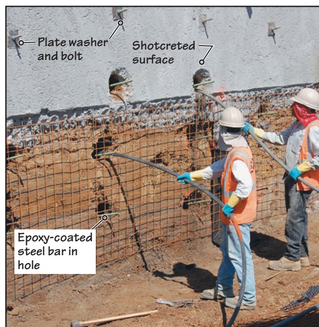
FIGURE 11.26 (a) Drilling of holes in excavated soil. (b) Grouting of holes after the epoxy-coated steel bar (soil nail) has been placed in the drilled holes.
