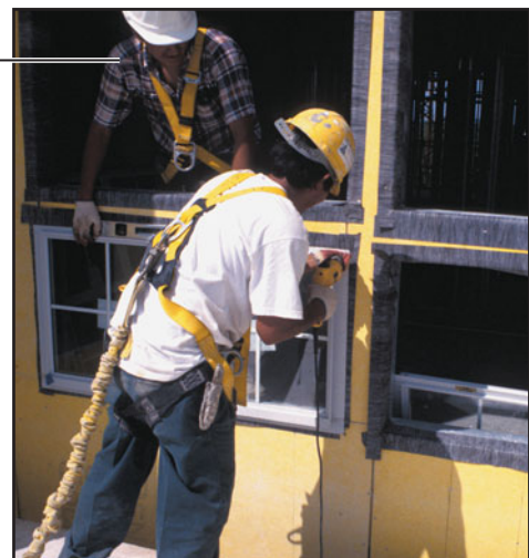
(b) Window being brought into the opening. Observe the self-adhering waterproof tape around the rough opening.
