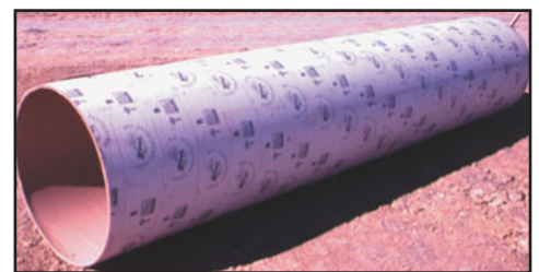
(b) One-time use fiberboard form for a round concrete column.
