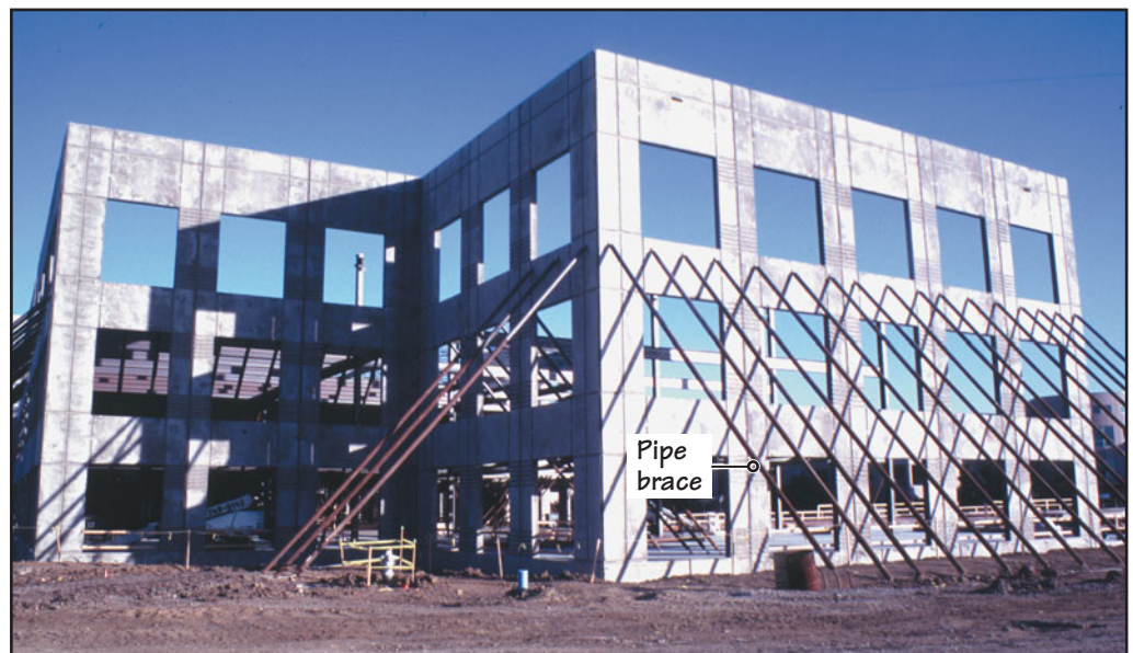
FIGURE 26.30 A typical tilt-up building consists of several wall panels, each extending from the foundation to the top. Pipe braces support the panels temporarily, and may be placed on the outside of the building (as shown here) or the inside of the building.
