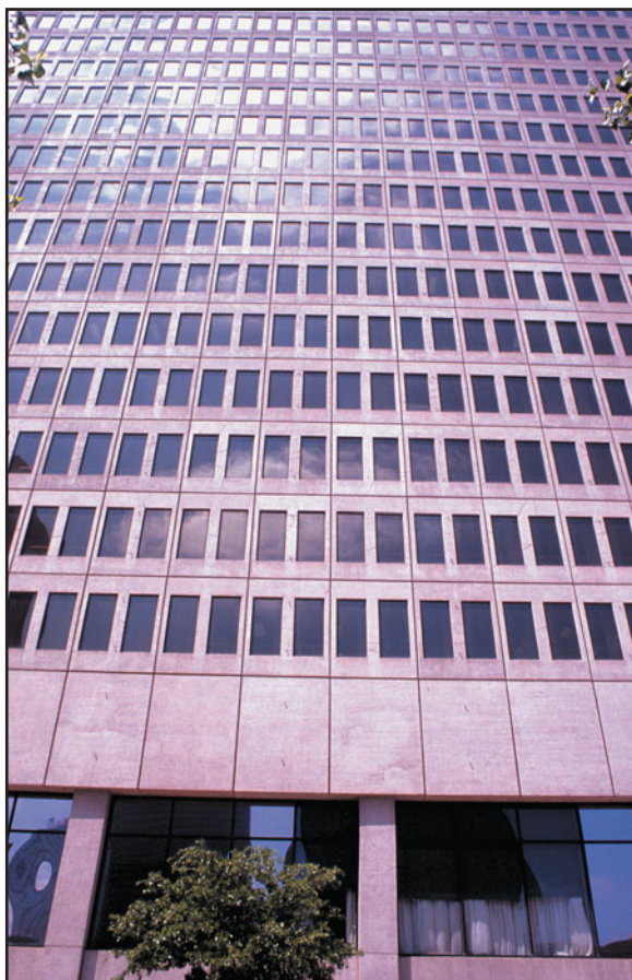
FIGURE 28.37 A typical office building with precast concrete curtain wall panels.
