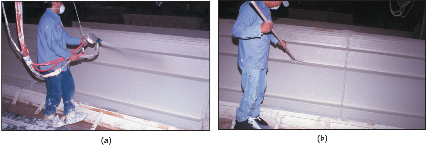
FIGURE 28.55 (a) Spraying of a GFRc mix over the mist coat. (b) Consolidating the GFRc mix using a roller around the bends, edges, and corners.
