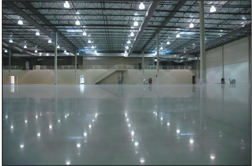
FIGURE 36.15 A concrete floor that has been highly polished with an abrasive medium. Notice the mirror-like reflection and the clarity of the reflected light fixtures. (Used with permission of the Concrete Polishing Association of America.)
