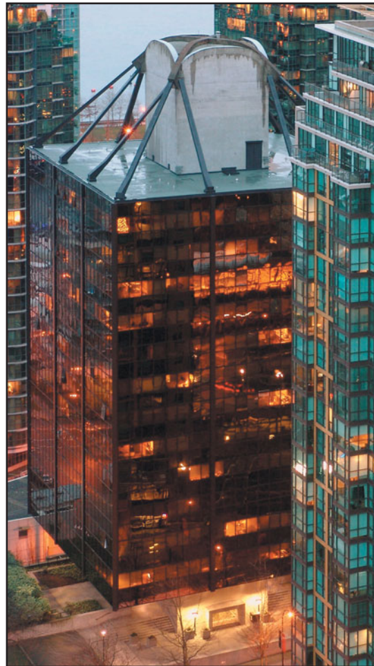
FIGURE 25 The 12-story West Coast Transmission Company Building, Vancouver, Canada, consisting of a reinforced concrete shear core. Note that there are no columns in the building, and the only support system is a reinforced concrete central core. The absence of columns gives a large, column-free space at the ground. The floors are framed out of steel wide-flange beams and are suspended at the perimeter from the core with steel cables. Similar buildings (with floors suspended from a concrete or steel-framed central core) have been constructed in several places [19.1]. (Photo by Alexander Ulyanov/Emporis)
