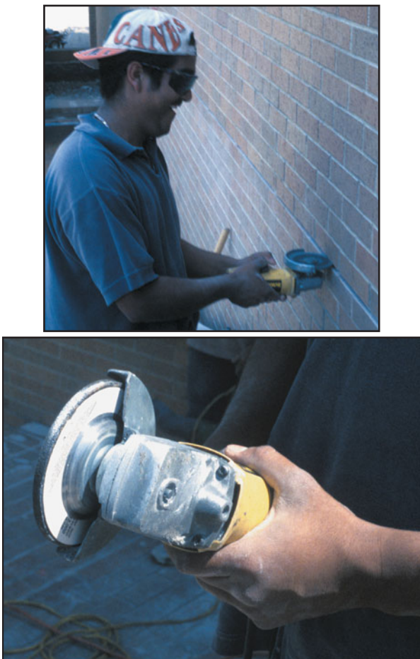
FIGURE 24.29 Grinding of mortar joints in preparation for repointing.
