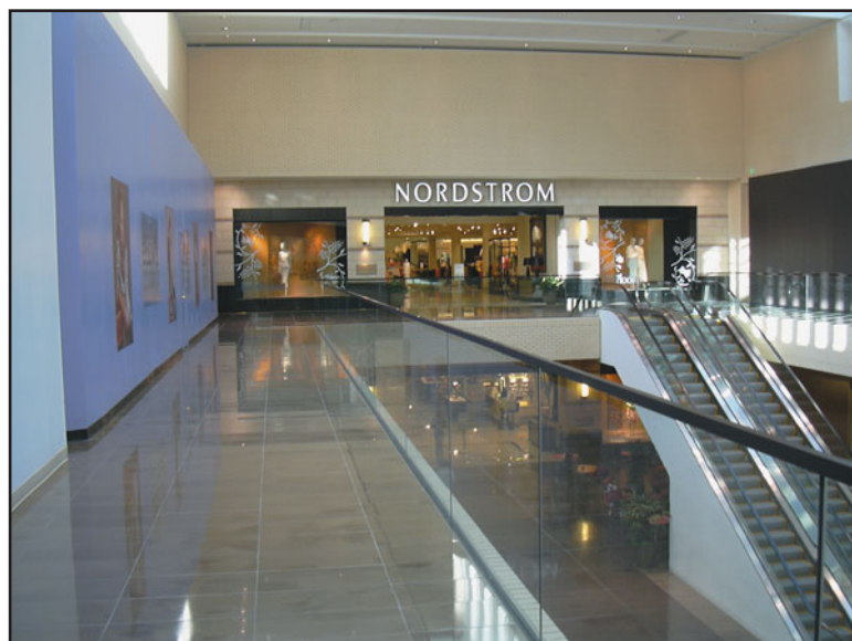
FIGURE 36.16 A clear coating applied to exposed concrete flooring. (Used with permission of RetroPlate System, PSI Permanent Surfaces; photo by Rhonda Clinton.)
