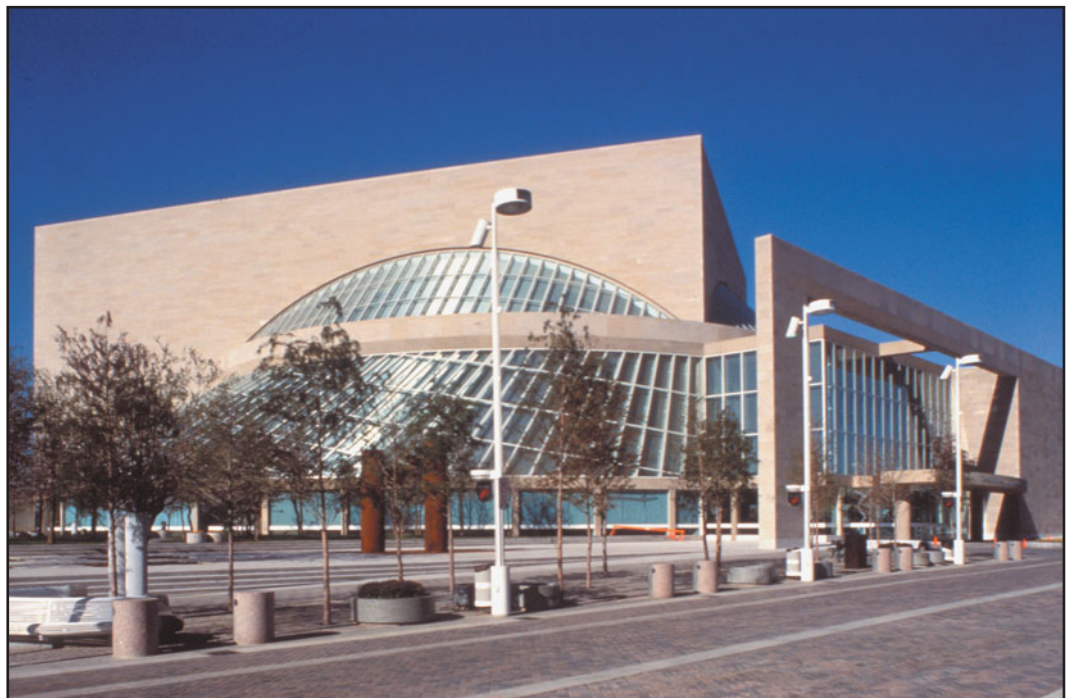
FIGURE 24.1 (b) Smooth-surfaced limestone cladding, Morton Meyerson Symphony Center, Dallas, Texas. Architect: I. M. Pei and Partners.
