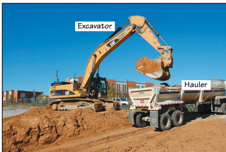
(a) Excavator and hauler
