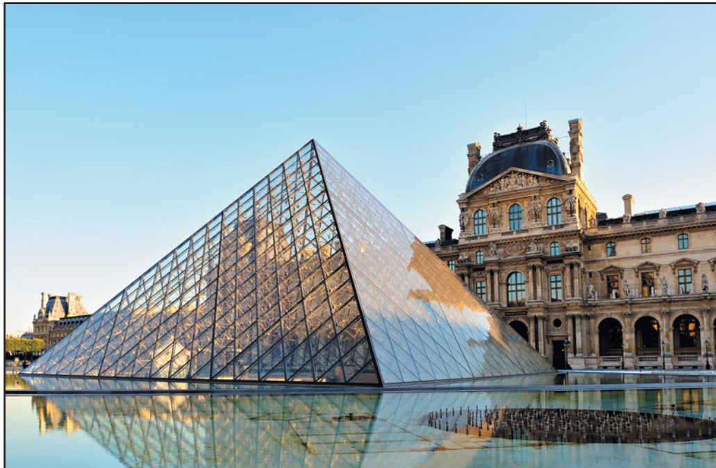
FIGURE 30.3 A large glass pyramid admits light into an underground addition to the Louvre museum, Paris, France. Architect: I. M. Pei and Partners. (Photo by Zoran Karapancev of Shutterstock)
