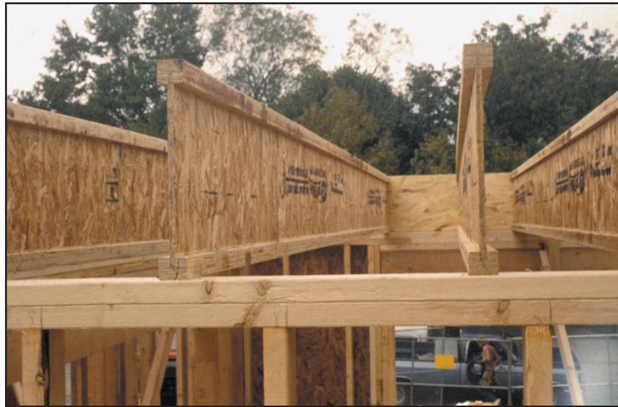
FIGURE 14.12 I-joists are commonly used as floor joists because of their greater dimensional stability and stiffness and their availability in longer lengths than solid sawn lumber joists.
