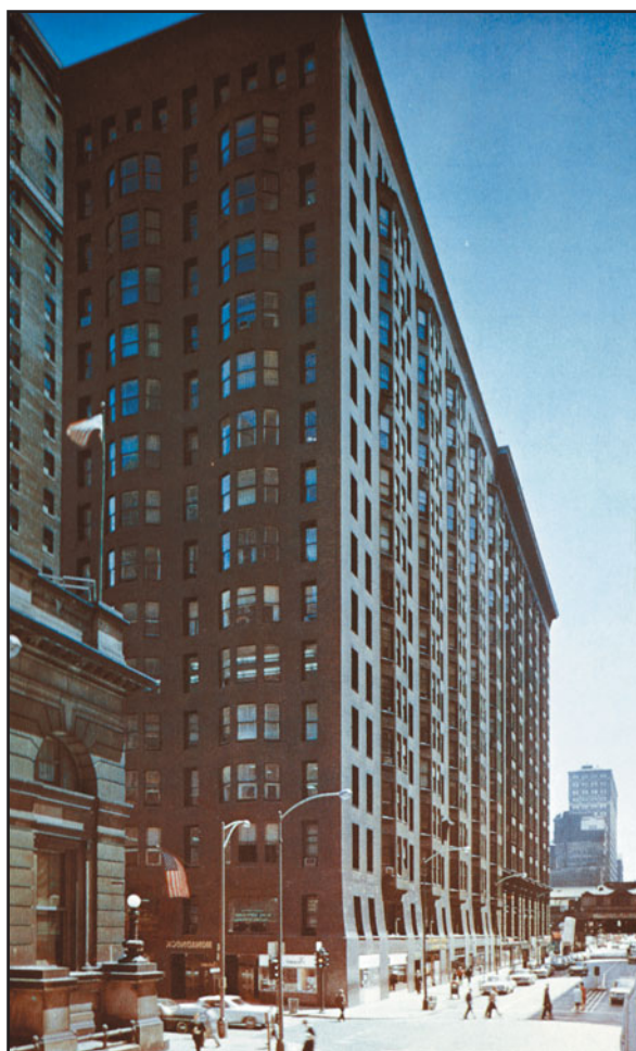
FIGURE 26.3 (a) In resisting wind loads, the exterior walls in historic load-bearing masonry buildings were designed as freestanding cantilevers. Therefore, the thickness of walls at lower floors increased substantially with an increase in the height of the building. (b) Monadnock Building, Chicago, completed in 1891, preserved as the last high-rise traditional bearing-wall structure. The walls at the ground floor are approximately 6 ft thick. Architects: Burnham and Root. (Photo courtesy of Dr. Jay Henry)
