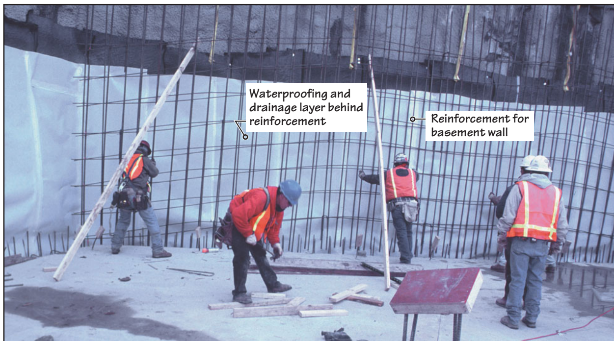
FIGURE 12.45 (a) In this deep basement, part of the cut face has been shotcreted. The shotcreted face is treated with waterproofing and a drainage mat layer. Additional shotcreting on the earth retention system will be done as construction of the reinforced concrete basement wall progresses. (b) After installation of waterproofing and the drainage mat, reinforcement is laid for the basement wall. This will be followed by wall formwork and concrete placement.
