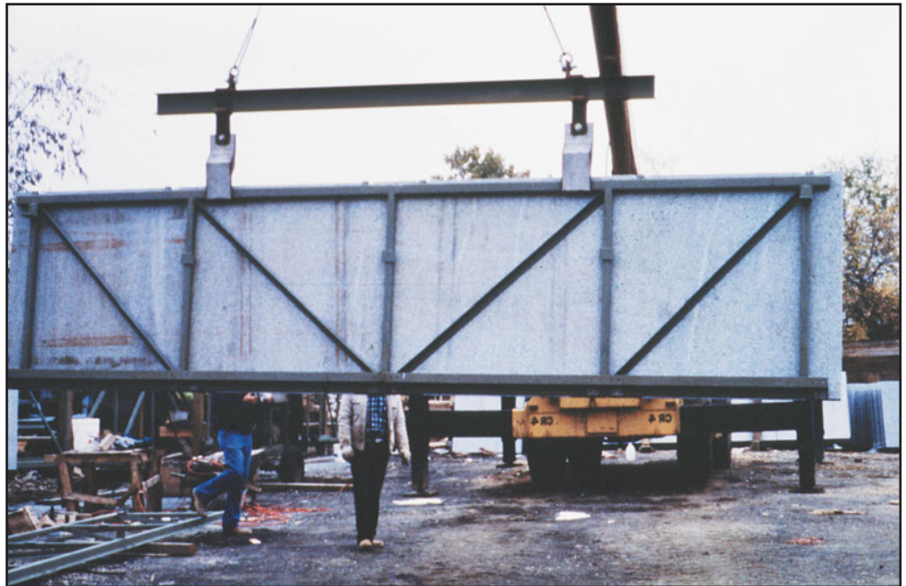
FIGURE 29.47 A prefabricated stone curtain wall panel. (Photo courtesy of Dee Brown, Inc.)
