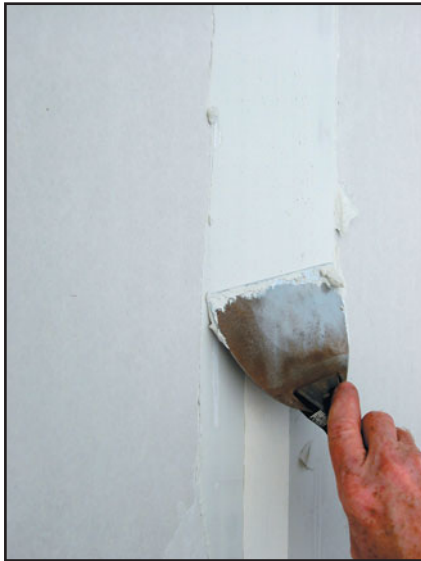
FIGURE 16.25 Joint compound filling over joint tape. (Photo courtesy of Tommy Eaton)
