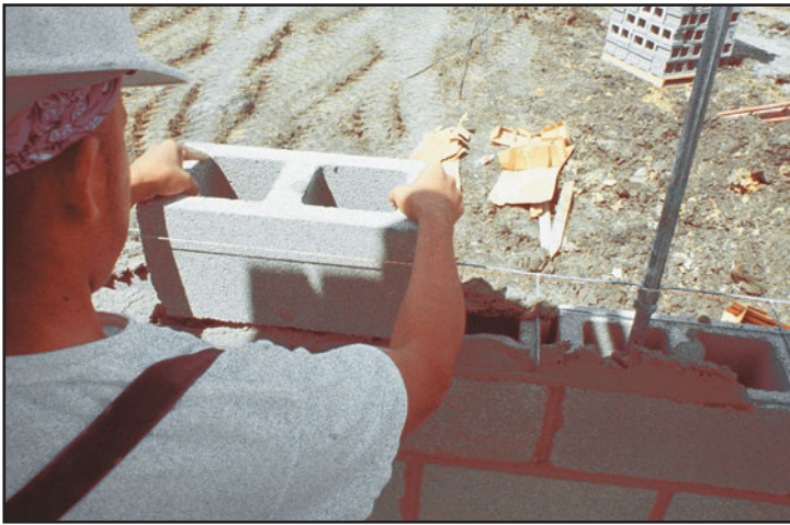
FIGURE 25.15 The laying of a CMU is a two-hand operation versus the one hand used in laying bricks.
