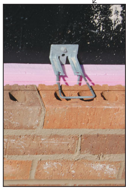
(c) A typical two-piece anchor consisting of a: (i) sheet metal anchor and (ii) wire anchor for reinforced-concrete backup members (walls, beams, and columns)
