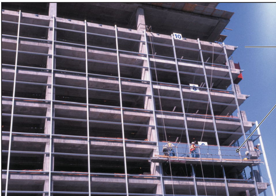
FIGURE 32.2 (a) The progress in the installation of a stick-built glass curtain wall on an office building in which the lower floors are parking floors and the upper floors are office floors. See also Figure 32.2(b).
