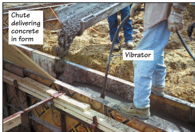
FIGURE 21.28 Consolidation of concrete using a power-driven vibrator.
