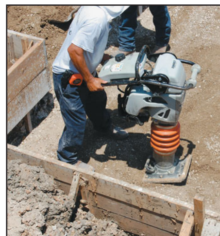
(d) Mini compactor (rammer), generally used for compacting small areas
