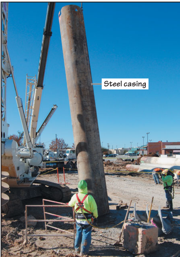
FIGURE 12.16 A steel casing being lowered into a pier hole.
