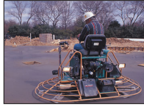
FIGURE 21.31 Troweling of concrete with a power-driven troweling machine, which is available in two different types, as shown. Each machine has metal blades that rotate over the concrete surface.
