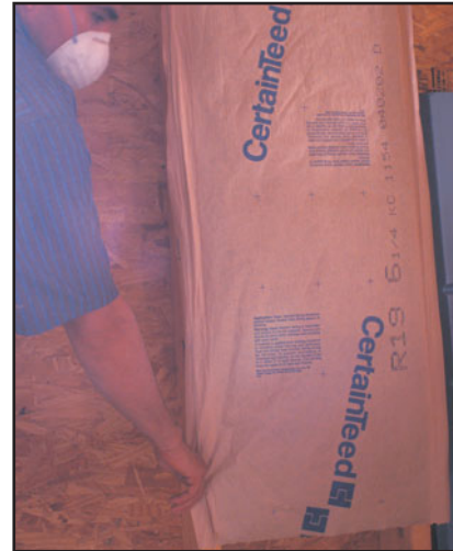
FIGURE 2(b) Kraft paper faced fiberglass insulation installed between studs. (Photo courtesy of CertainTeed Corporation)
