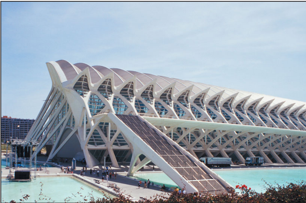
FIGURE 21.11 (b) Concrete structural frame work in the City of Arts and Sciences, Valencia, Spain, by architect-engineer Santiago Calatrava, illustrating the sculptural properties of concrete.
