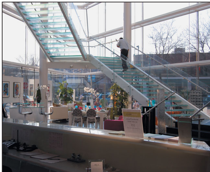
FIGURE 35.1 Images showing the aesthetic potential of stairs; see also Figure 35.20. (a) An entrance lobby stair with structural steel beams (stringers) and concrete-filled sheet-steel tread pans (see Figure 35.13). (b) A highly transparent glass wall showcasing the stair in the Madison Museum of Contemporary Art, Madison, Wisconsin. (c) Stair in the entrance lobby of the Madison Museum of Contemporary Art, Madison, Wisconsin with structural steel beams (stringers) and glass treads. Architect: Cesar Pelli and Associates.
