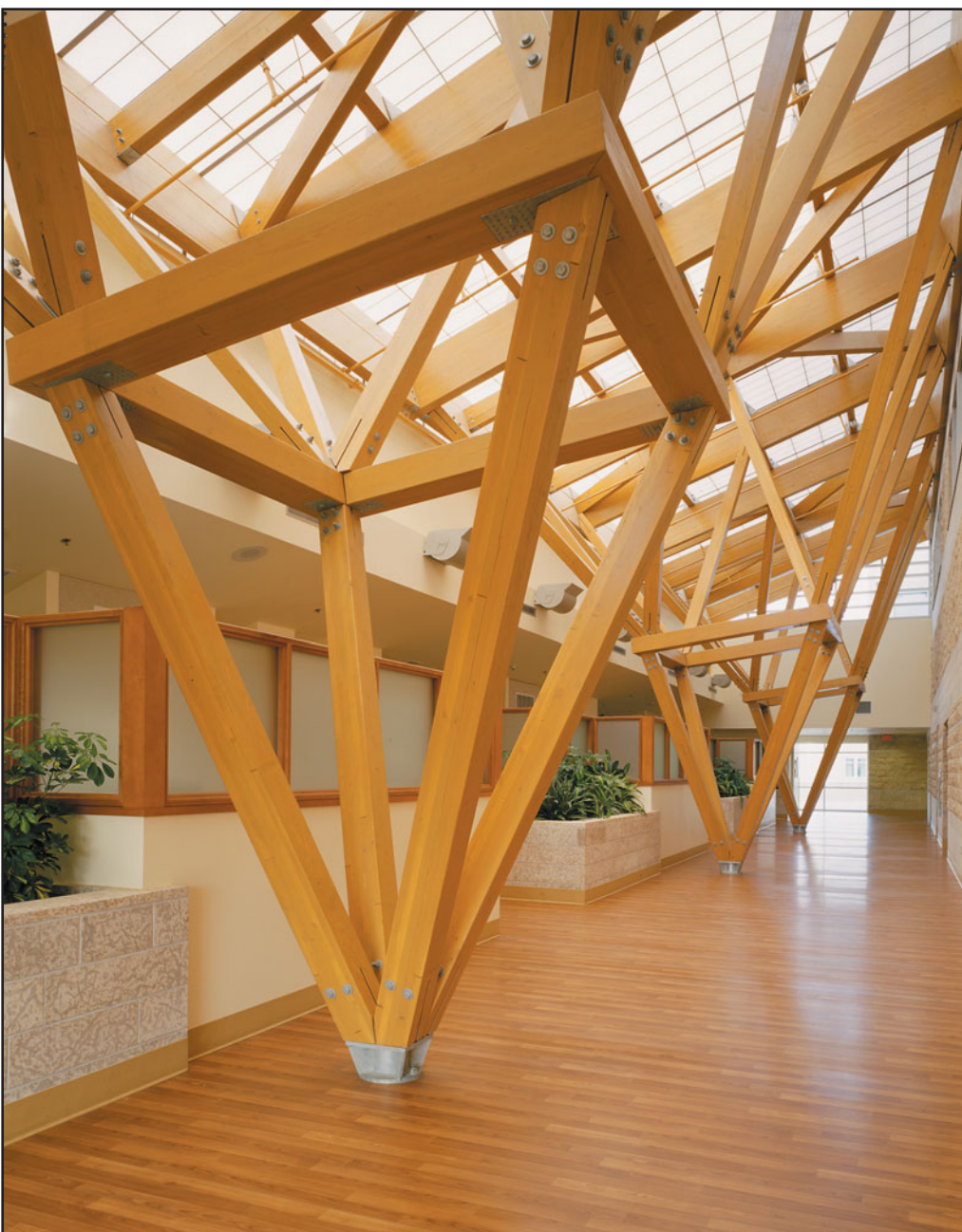
FIGURE 13.4 Wood-framed skylight in the Thunder Bay Regional Health Sciences Centre, Thunder Bay, Ontario, Canada, by Salter Farrow Pilon Architects (Farrow Partnership Architects; Salter Pilon Architects successors). (Photo: Peter Sellar Klik photography, provided courtesy of Farrow Partnership Architects Inc.)
