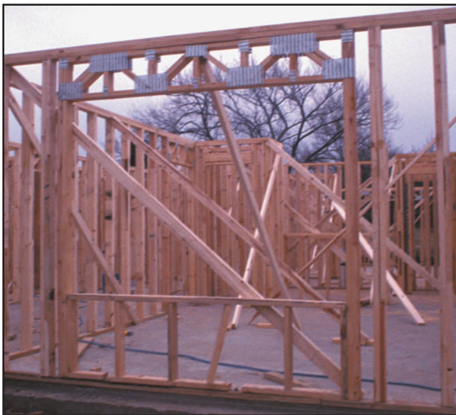
FIGURE 14.20 Trussed lintel over an opening.
