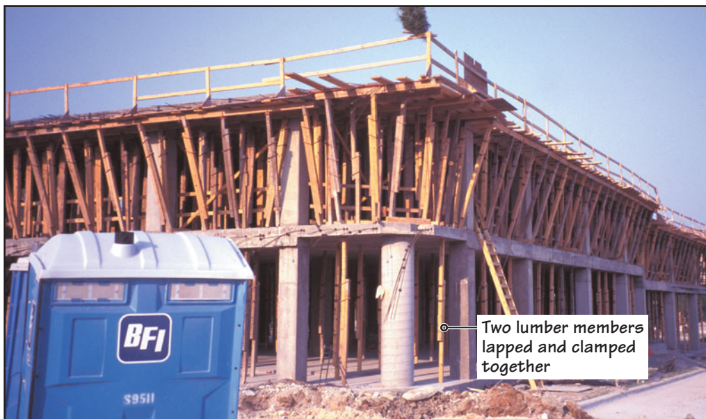
FIGURE 22.6 Shores for a reinforced-concrete floor slab in which two dimension lumber members are lapped and clamped together with a patented device. The lapped and clamped assembly provides adjustment in the height of a shore.
