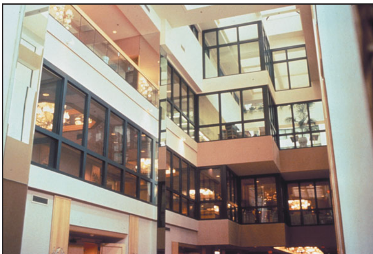
FIGURE 30.28 Lobby at the Red Lion Inn, Costa Mesa, California. Glazed walls provide a 1\frac{1}{2} -h fire rating. (Photo courtesy of SAFTI FIRST, a division, O’Keeffe’s Inc.)
