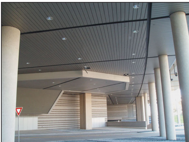
FIGURE 37.13 A suspended linear metal ceiling in an area where streets and drives pass under a building.
