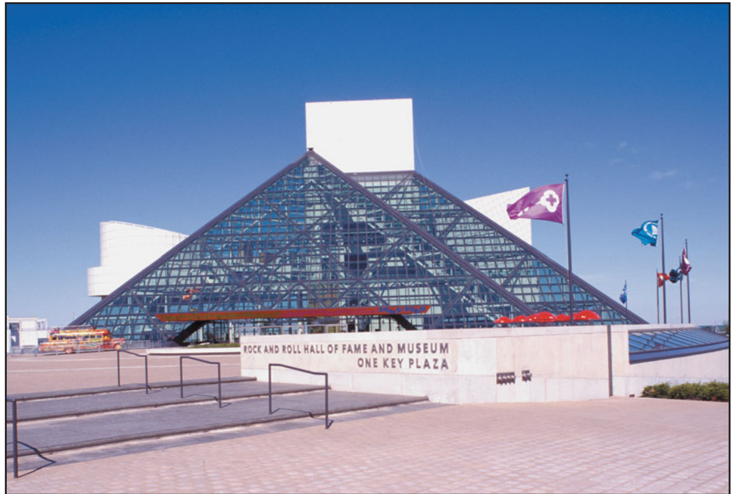
FIGURE 18.1 Rock and Roll Hall of Fame and Museum, Cleveland, Ohio. The sloping glass skin framed with tubular steel trusses spans nearly 200 feet. The steel tower structure is seen in the background. Architects: Pei, Cobb, Freed and Partners. (Photo courtesy of Dr. Jay Henry)
