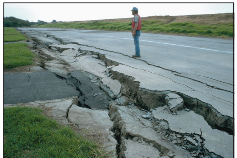
FIGURE 3.17 Fissures in the ground caused by the 1989 Loma Prieta earthquake, San Francisco Bay area (Richter magnitude 7.0). (Photo obtained from the World Wide Web using the following URL: http://pubs.usgs.gov/dds/dds-29/tif/img0087.tif )
