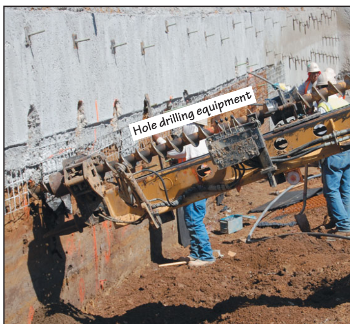
FIGURE 11.26 (a) Drilling of holes in excavated soil. (b) Grouting of holes after the epoxy-coated steel bar (soil nail) has been placed in the drilled holes.
