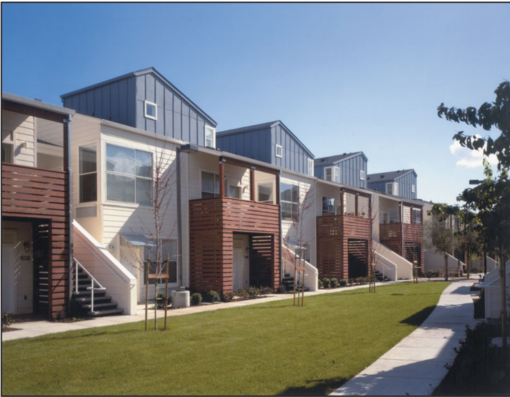
FIGURE 13.3 Montage Apartments in Palo Alto, California, by Seidel/Holzman Architects, constructed of wood light frame and clad in combination of fiber-cement lap, fiber-cement panel, and cedar batten siding. (Photo courtesy of Tom Rider)
