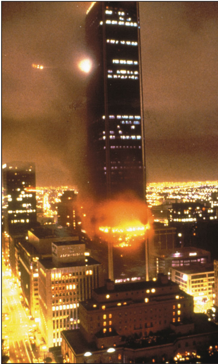
FIGURE 7.1 Four floors of the First Interstate Building in Los Angeles, California, gutted with fire. The building is still standing and is in service. Its survival is ascribed primarily to its fire-safe construction. (Photos courtesy of W.R. Grace & Co. Both photos are copyrighted by W.R. Grace & Co.)
