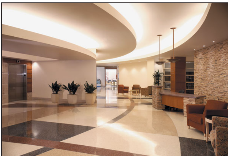
FIGURE 36.8 The creative use of divider strips and colored terrazzo at the entry of a hospital. (Photo courtesy of HKS Inc.)
