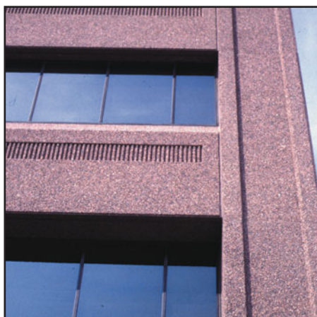
FIGURE 28.39 (c) Panel with an exposed aggregate finish.
