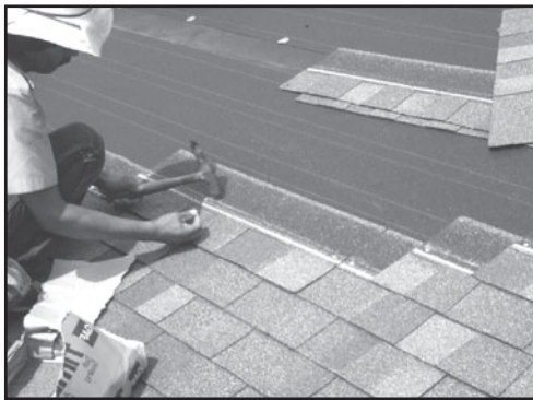
FIGURE 16 Application of roof felt underlayment. An asphalt-treated felt (called roof underlayment ) is laid over the roof sheathing (deck) before it is covered with roof shingles. The felt functions as the second line of defense against water penetration, the first line of defense being the shingles; see Chapter 34.
