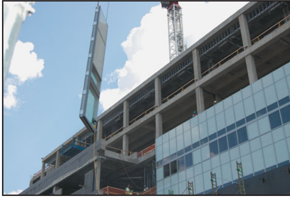
(a) Using a crane, unitized curtain wall elements are carried up from the delivery truck to the building facade
