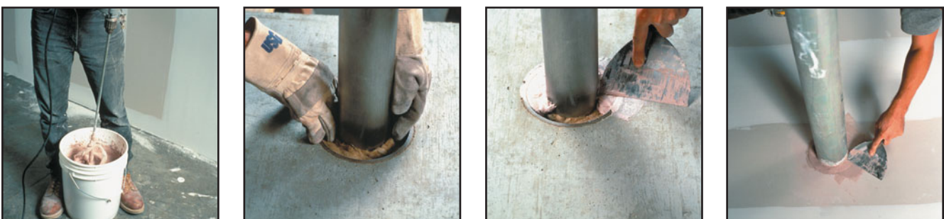
FIGURE 7.13 A typical fire-stopping around a penetration in a floor generally consists of high-density mineral wool pressure fitted into the void, followed by a semiliquid, fire-resistant sealant troweled over mineral wool packing. (Photo courtesy of U.S. Gypsum Company)
