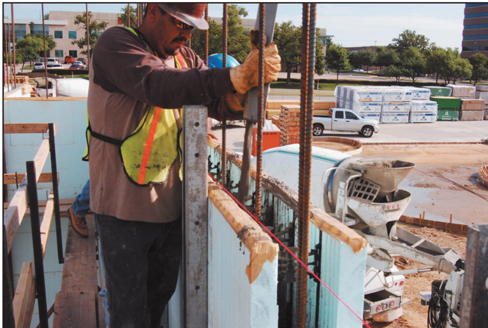
(b) Concrete being placed in an ICF wall
