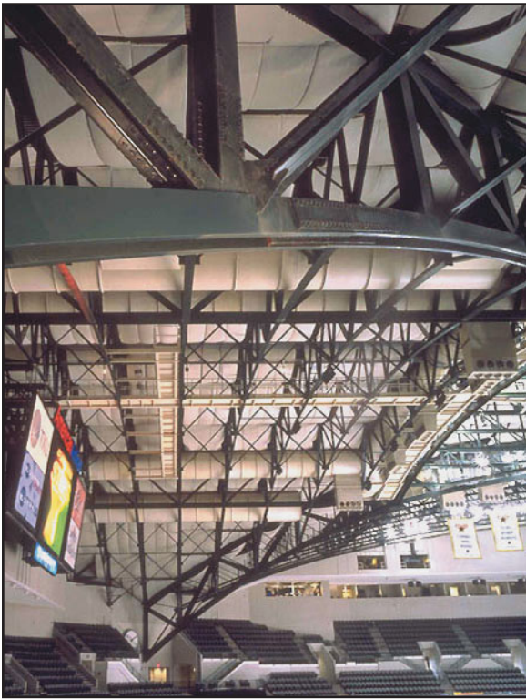
FIGURE 37.3 The building structure, utilities, and lapidaries of a professional basketball and hockey stadium are exposed as part of the architectural design. (Photo courtesy of HKS Inc.)
