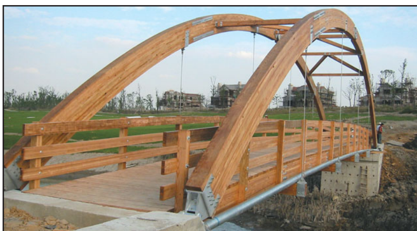
FIGURE 14.6 Seshan Golf Course bridge near Shanghai, China. (Photo courtesy of APA—The Engineered Wood Association)
