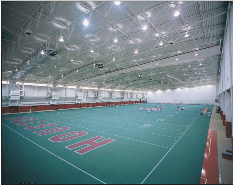
FIGURE 27 The use of steel trusses in the University of Houston Athletic Center (truss span is approximately 200 ft; truss depth is approximately 10 ft at midspan). (Photo courtesy of Nucor-Vulcraft Group)
