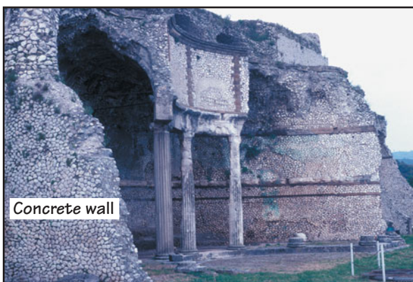
FIGURE 21.3 Temple at Palestrina, Italy, built around the first century BC, showing concrete walls. In this temple, the facing stone veneer, used as permanent formwork for the concrete walls, has disintegrated and disappeared. (Photo courtesy of Professor Michael Yardley)
