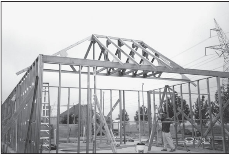
FIGURE 20.25 Use of CFS roof trusses. (Photo courtesy of American Residential Steel Technologies)
