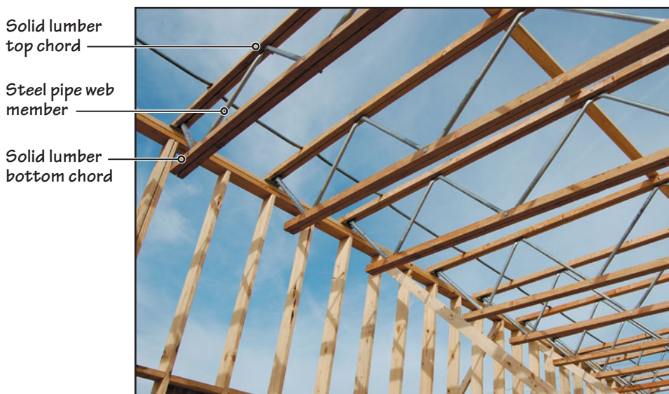
FIGURE 14.22 Wood-steel trussed joists.
