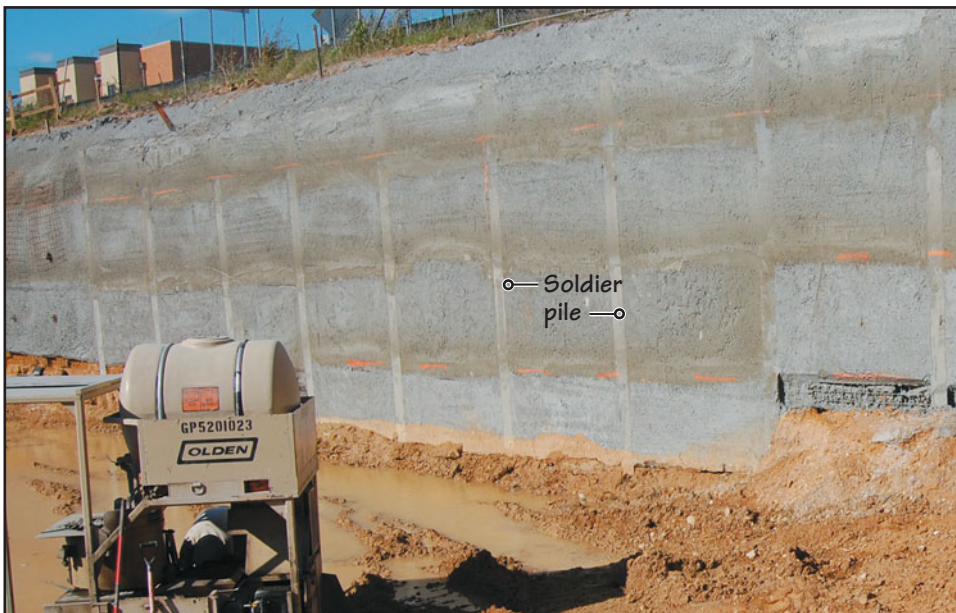
FIGURE 11.16 Excavation support using cantilevered soldier piles.
