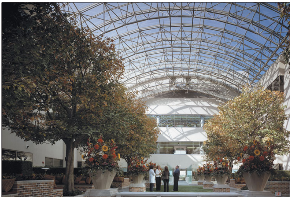
FIGURE 30 Arched steel space frame used in the atrium of William Beaumont Hospital, Royal Oak, Michigan. (Photo courtesy of Novum Structures, Inc.)
