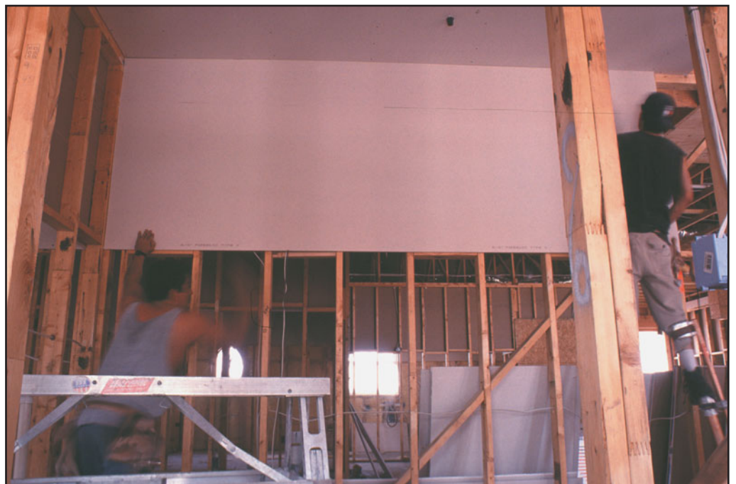
FIGURE 16.23 Gypsum board panels for ceilings are typically attached prior to wall panels.
