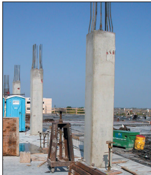
FIGURE 22.21 Column bars bent inward to receive bars for the upper floor.
