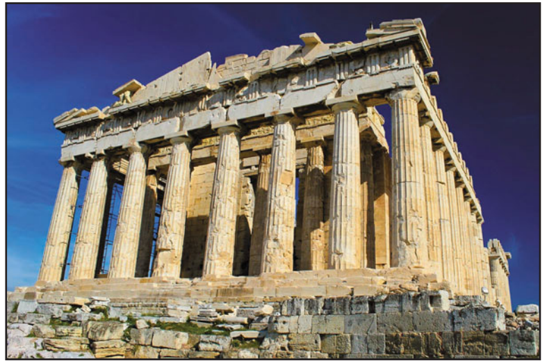
FIGURE 4.1 Parthenon, Acropolis, Greece. Observe the relatively small span of beams in response to the weakness of stone in bending. (Photo by Brent Wong/Shutterstock)
