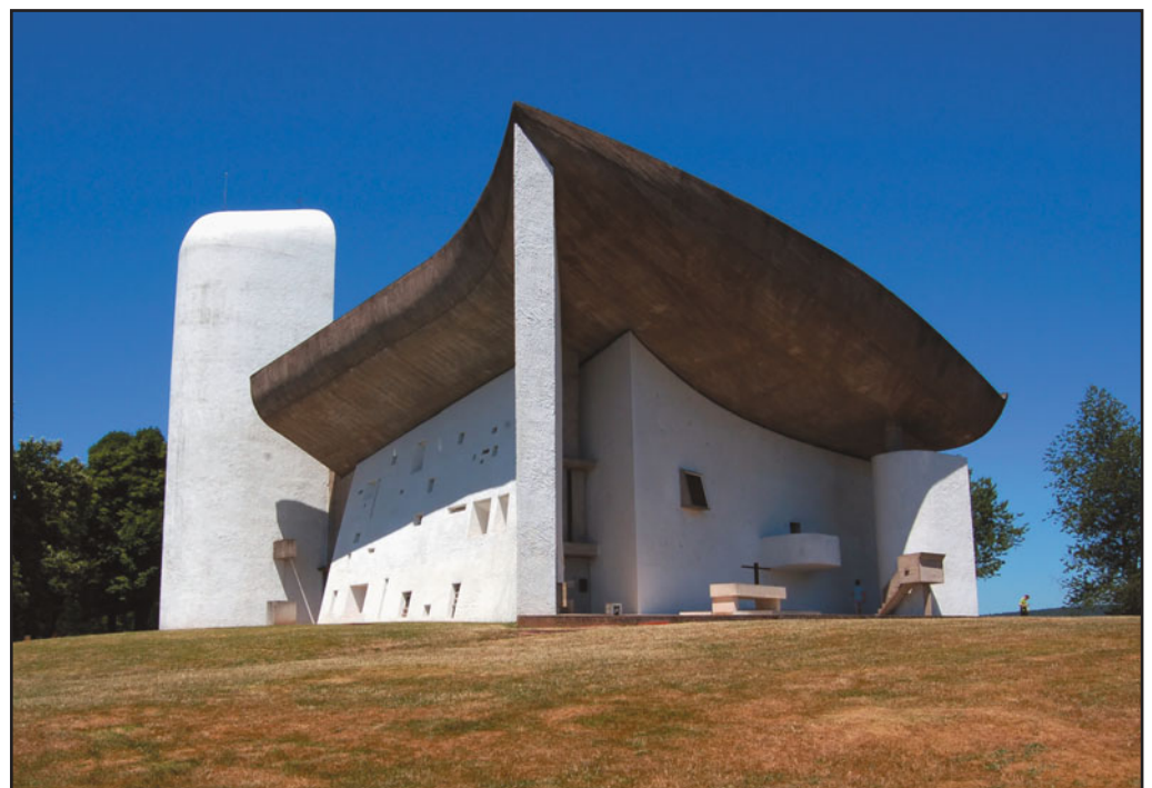
FIGURE 21.11 (a) Chapel at Ronchamp, France, by architect Le Corbusier. Le Corbusier was among the pioneers in exploiting the sculptural properties of concrete in building structures. (Photo by Lazar Mihai-Bogdan/Shutterstock)
