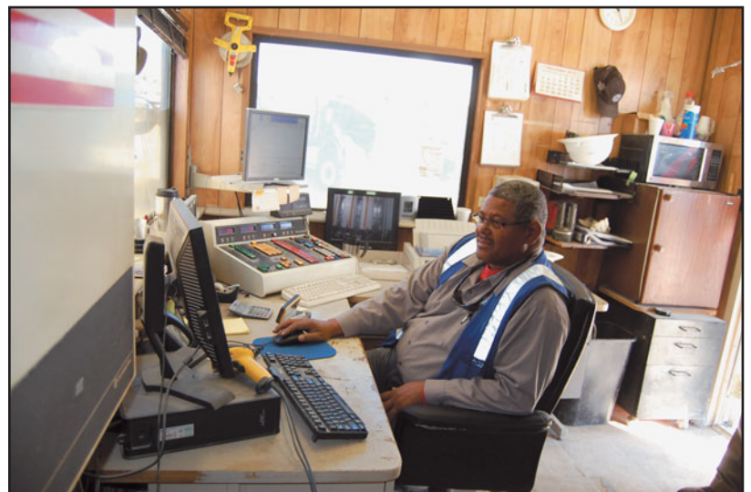
FIGURE 21.23 A typical control room in a ready-mix plant.
