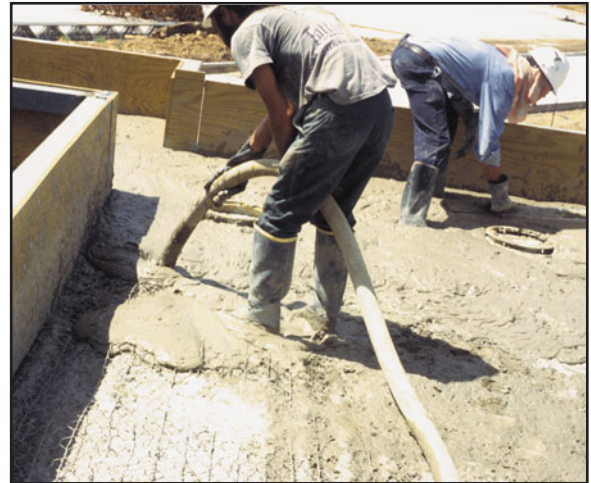
FIGURE 10 Insulating concrete being poured over a roof deck.
