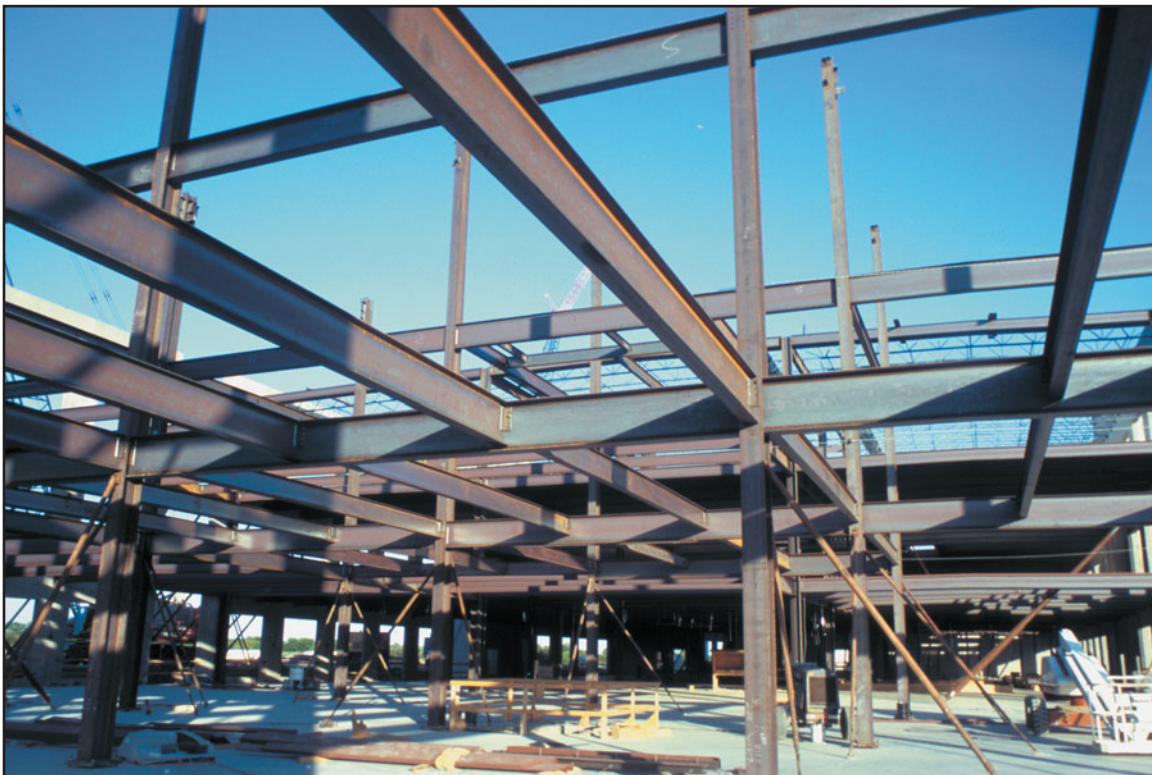
FIGURE 18.11 A steel building under construction has the appearance of a skeleton. Therefore, when steel buildings first appeared in Chicago toward the end of the nineteenth century, the terms skeleton cage , steel skeleton , and skeleton frame were coined to describe their appearance.
