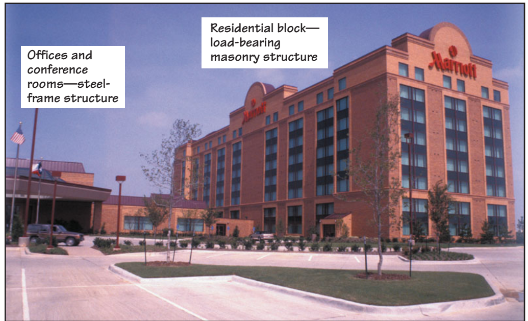
FIGURE 26.23 (f) The eight-story hotel residential block with a masonry bearing wall structure (shown under construction in (a) to (e)). The office and conference areas in this building are in steel frame because of their large, unobstructed spaces.
