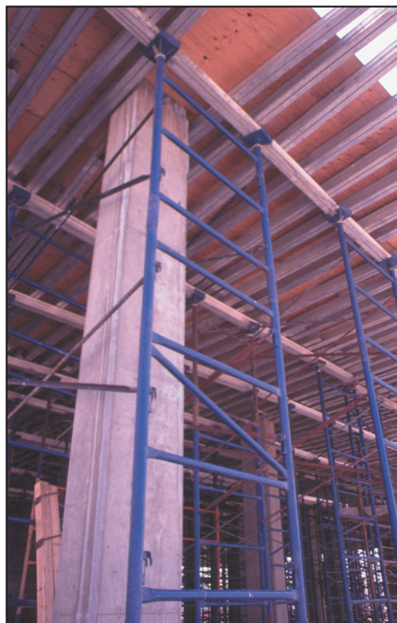
FIGURE 22.8 Steel pipe scaffold shores are available in panel frames in widths of 2 to 5 ft and heights of 4 to 6 ft. Panel frames can be assembled vertically and braced diagonally to make a stable shore frame.
