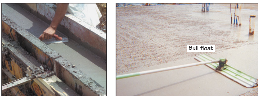
FIGURE 21.30 Floating of a small concrete surface with a hand float and a large surface with a long-handle bull float.
