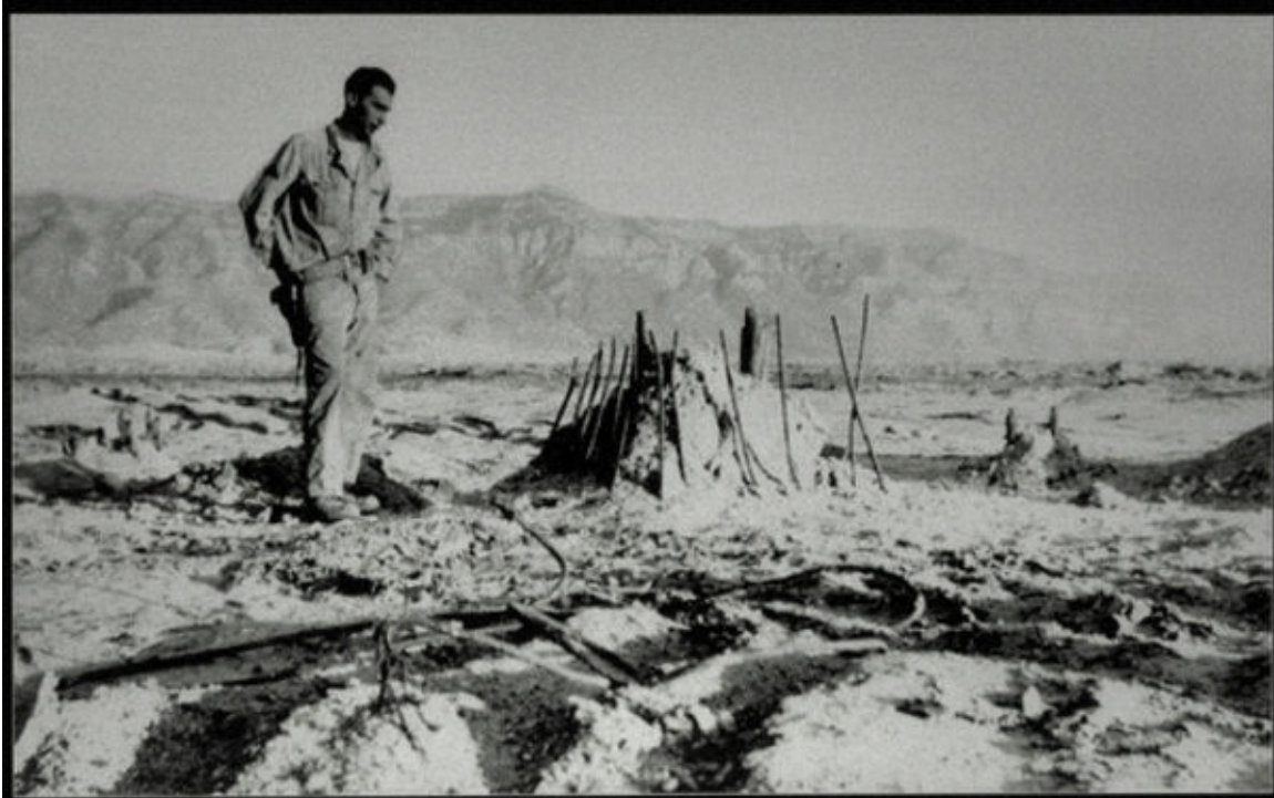
A soldier examines one of the footings to the 100-foot steel tower at ground zero months after the test.
