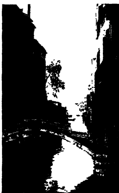
A BRIDGE WITHOUT A PARAPET
