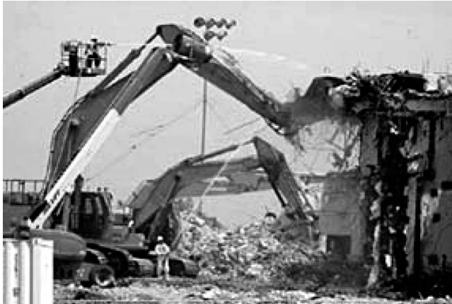
FIGURE 18.10 Typical large equipment demo.
