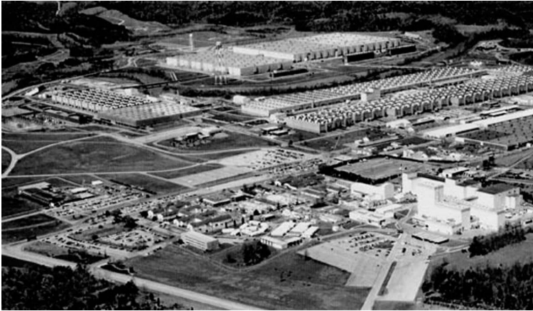
FIGURE 12.5 Oak Ridge Gaseous Diffusion Plant in Oak Ridge, Tennessee.
