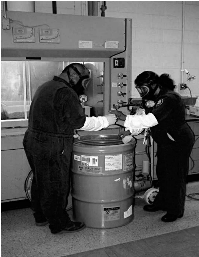
FIGURE 18.8 D&D work in front of equipment with PPE.
