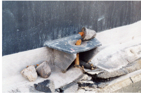
(b) Cut off of anchor bolt
